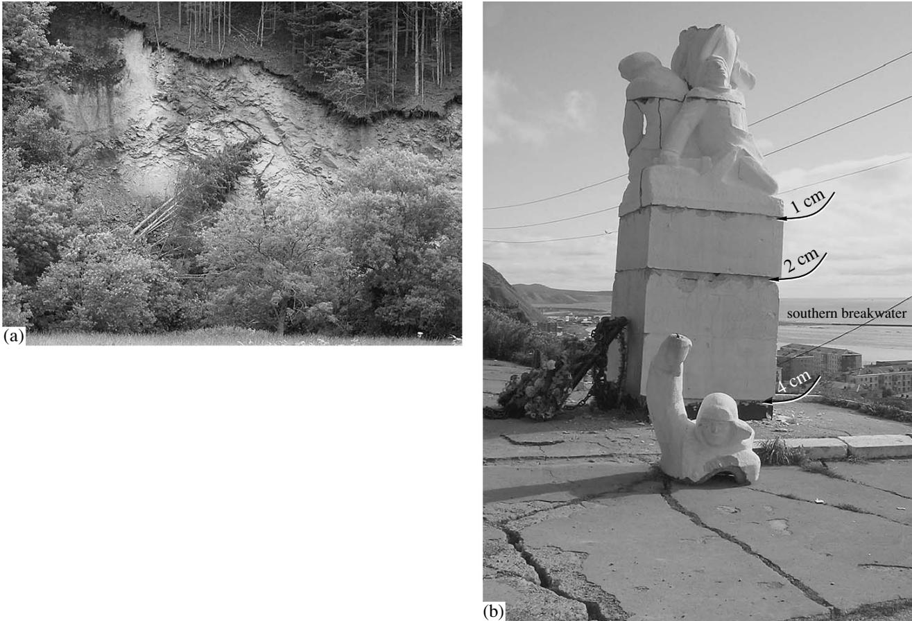
**Fig. 5.** Landslide on the mountainous forested slope near the Lopatino settlement south of Nevelsk (a) caused by the double impact of the main shock and the strong aftershock (according to the observations of eyewitnesses); the monument to lost seamen (view from the northeast) (b).
