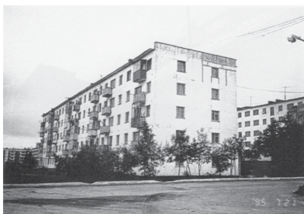
Fig. 1. Large concrete block construction 447C type in Okha.
